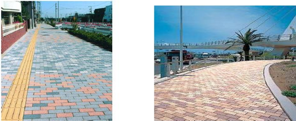
Figure2. Examples of Photocatalysts concrete unit pavers in Japan. (Source: Adnan et al. 2018)
