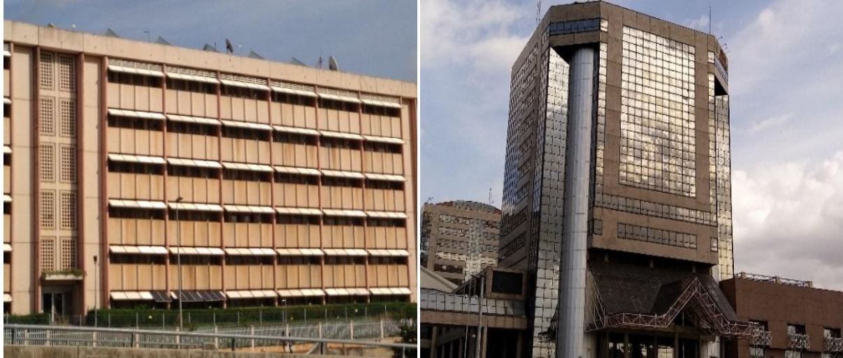
Figure 1. Dirt and water marks on the offices buildings in Nigeria.
